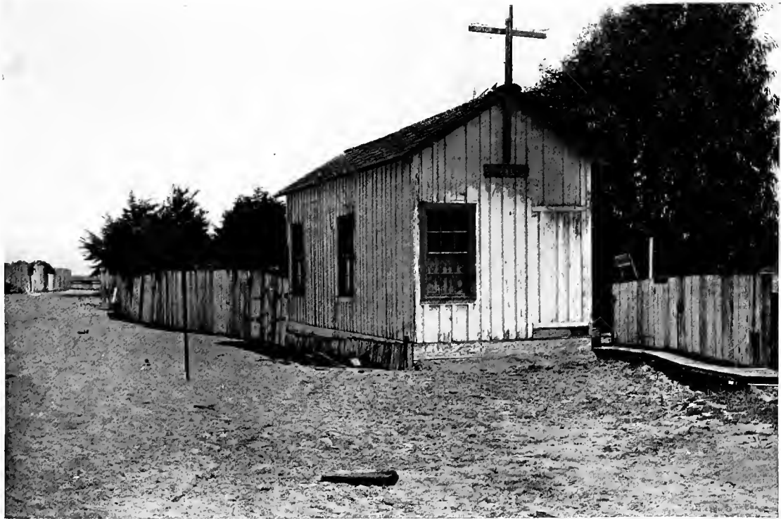
A. Moss Landing. House, tree, and fence moved 12 feet by lurching of ground toward Salinas River. A. C. L.
